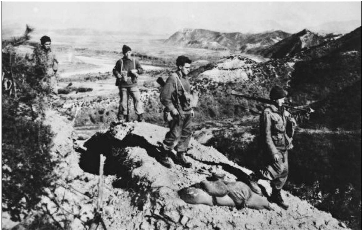
Men of B Company, 2 RAR, moving down off the Kansas Line to the battalion area after a week spent constructing defensive positions, 10 January 1954. AWM 157821
