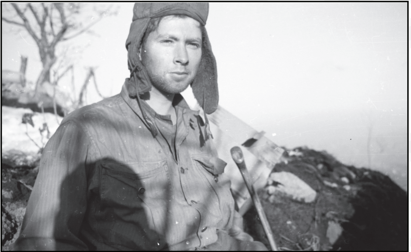
Peter Doyle chopping wood for bunker construction - Punchbowl - December 1951
